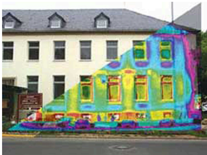
FIGURE 14.27 A thermograph of part of a building shows temperature variations, indicating where heat transfer to the outside is most severe. Windows are a major region of heat transfer to the outside of homes. (credit: U.S. Army)
